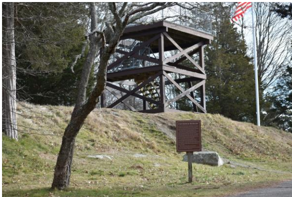
Photo: The steep slopes of the fort rise above the surrounding hilltop grade.
