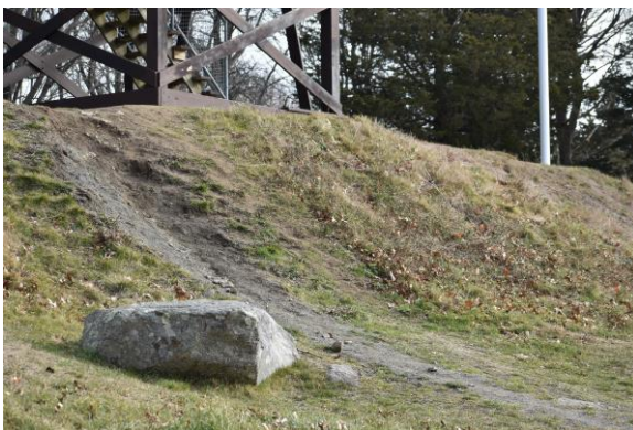
Photo: Eroded desire lines indicate where visitors have climbed over the earthworks to get to the observation tower.
